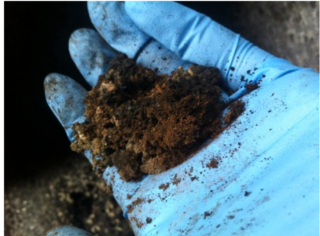
Fig 4. Light and malleable debris that can easily be removed from the duct by hand is a better potential sample.
