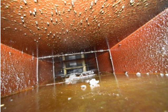
Fig 1. Liquid residue build-up.
